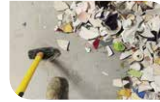
Project Break Smash Room Saturday 1st July
